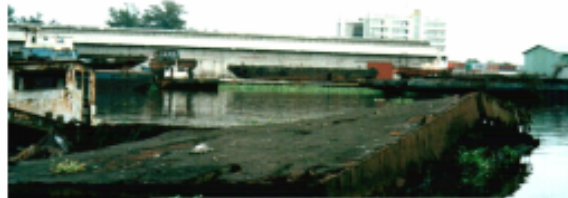
Wrecks: Environmental degradation
