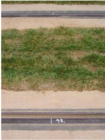
Figure 4: Rail marking on site.
