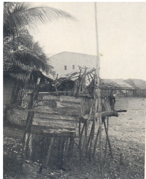
Typical Pit latrine
