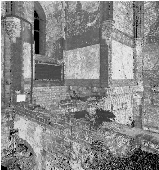
Figure 3. Raw gray scale coded point cloud
