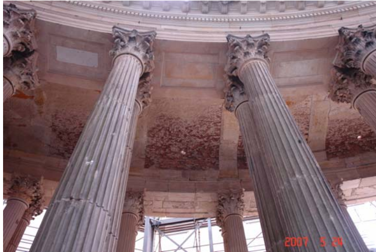
Figure 10. Actual conditions of the structure
