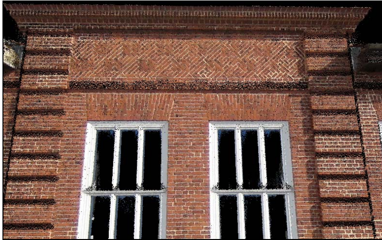
Figure 1. Coloured point cloud of the facade
