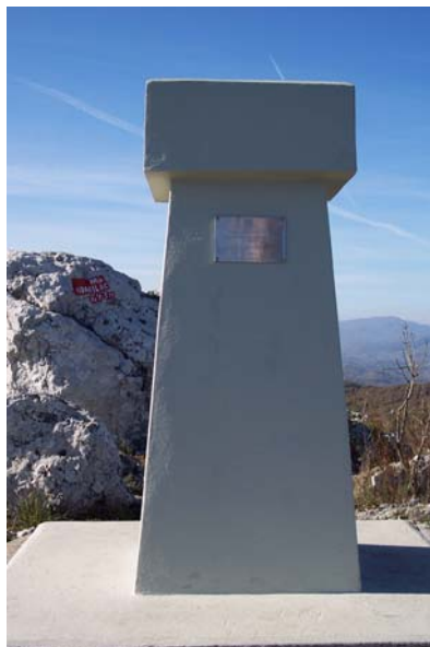
Figure 5. Renewed geodetic pillar
