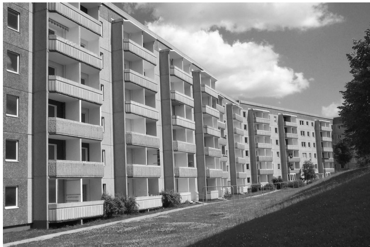
Figure 6: Large panel housing estates in the Dürer Quarter, a typical building style of the DDR.
