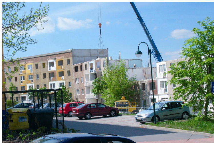
Figure 7: Running demolition of a housing estate.
