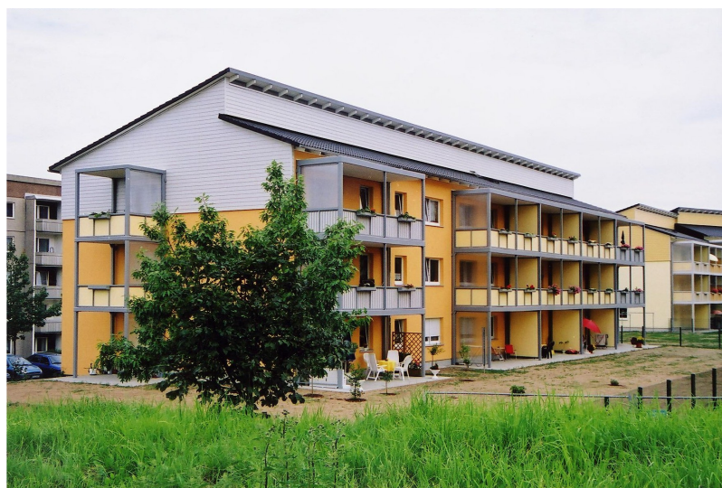
Figure 9: The Dürer Quarter after partial building demolition.
