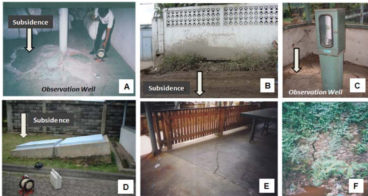
Figure 6. Examples of subsidence features in Bandung basin, adapted from Ruchijat (2006). In this Figure A: Ground lowering in the Rancaekek area (around RCK2 GPS stations); B and F: Hanging wall and structural cracking in the Leuwigajah area (around CMHI GPS station); C: Ground lowering in the Ujungberung area (around UJBR GPS station); D: Differential subsidence in the Gedebage area (around GDBG GPS station); E: Structural cracking around DYHK GPS station.
