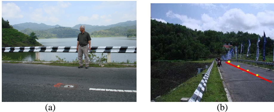
Fig.5. (a) Crest of Sermo dam where points monitor (prisms with yellow color) have been installed.
