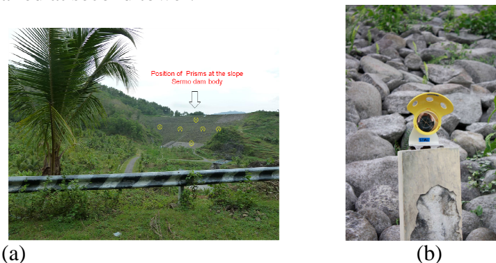
Fig.6. Target of monitoring with prism at slope of Sermo dam body
