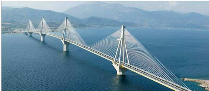
The Rion-Antrion Bridge, a SMART bridge.
