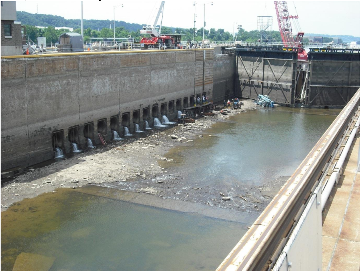
Figure 5 - Gate Monoliths to bedrock
