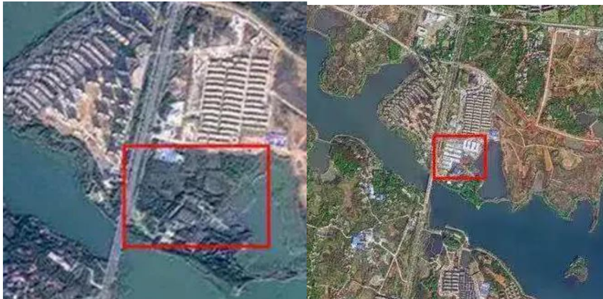
Fig. 9 Gaofen-2 and Jilin-1 multispectral satellite images showing the construction site of the Houshenshan hospital before and after construction.
