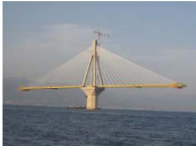
Figure 10 : Rion-Antirion Bridge in Greece (Marchetti et.al. 2004) - Basic construction of pylons - Cantilever construction
