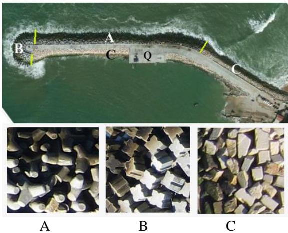
Fig. 14 Ericeira breakwater. Division related with the types of blocks of the armour layer (from Henriques et. al 2016)
