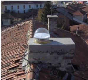
Fig. 7: Type 1 – Pedestal on the concrete base
