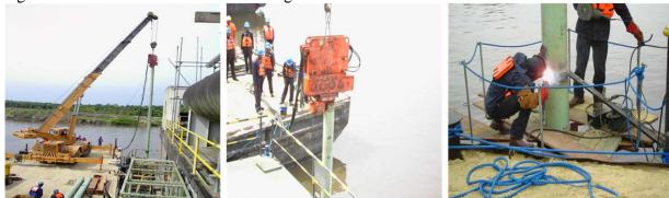
Installation of 16nos 12" double length Piles using vibro pile hamper and Welding work at the EPS barge location
