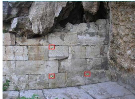
**Figure 3:** Example of monitoring points
