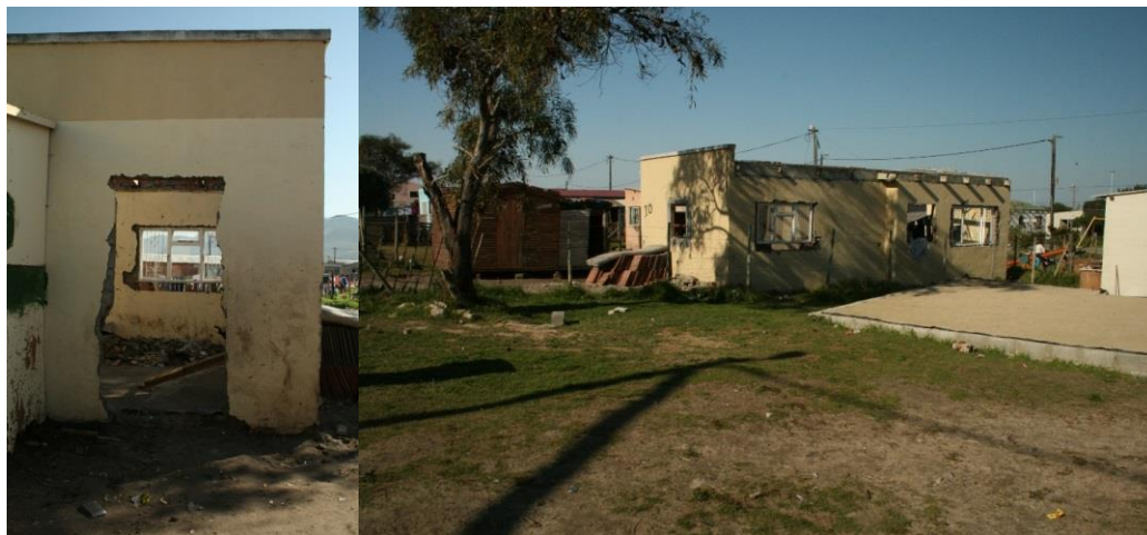
Figure 1 The Yellow House with Doors and Windows Removed from Extensions
