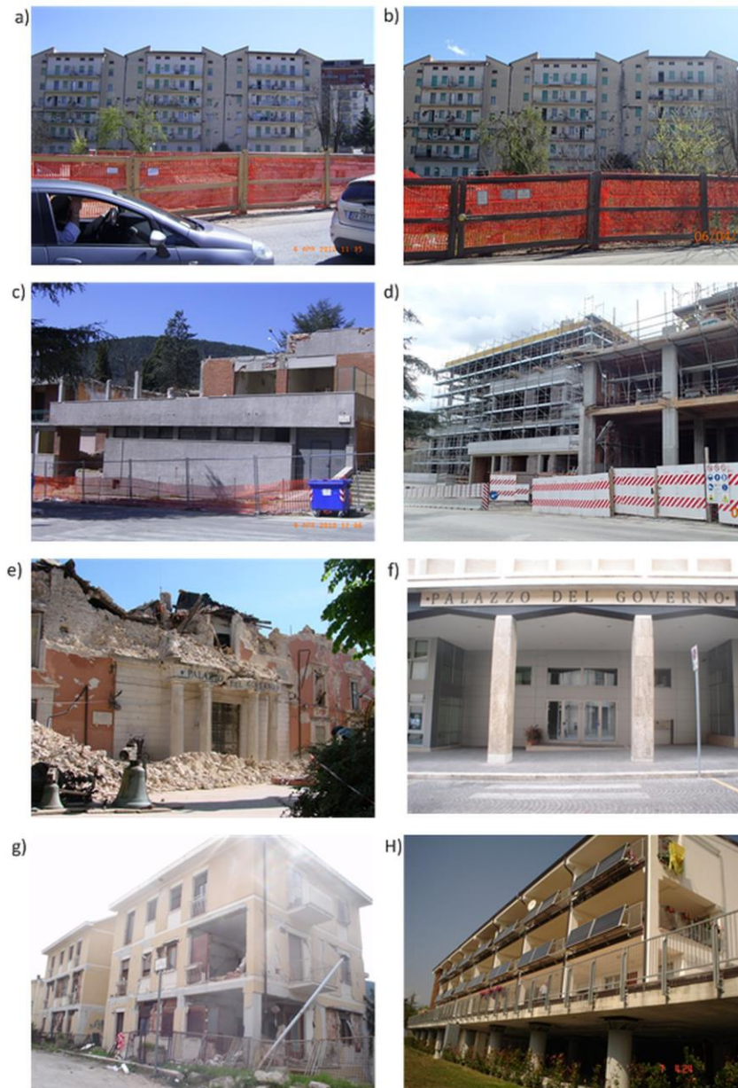
Figure 4. a) Buildings along via XX Settembre in 2010 (one year after the earthquake); b) buildings along via XX Settembre in 2014 (five years after the earthquake); c) building on viale Crispi in 2010; d) building on viale Crispi in 2014; e) government palace in 2009 (Photo: David Alexander); f) government palace relocated (2014) (Photos: Diana Contreras).
