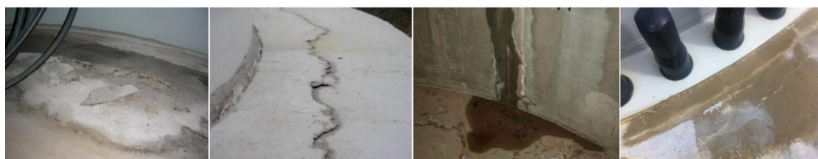
Spalling inside
