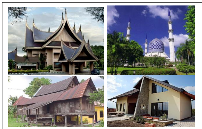
Figure 9: Top Left: A multilevel roof commercial building inspired by Rumah Minangkabau ; Top Right: Sultan Abdul Samad Mosque with tall pillars; Down Left: A kampung house in the city with usable attics; Down Right: A semidetached house with usable attic
