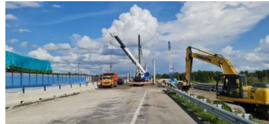
Reconstruction Sodong Bridge, Sept 2022
