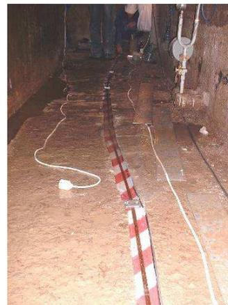
Figure 8: SMARTape installation in the inspection gallery.
