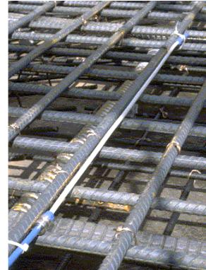
Figure 2: SOFO Sensor installed on a rebar
