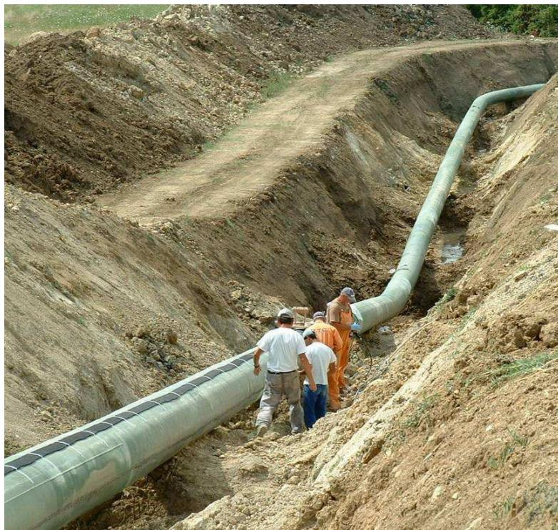
Figure 9: SMARTape on the gas pipeline.
