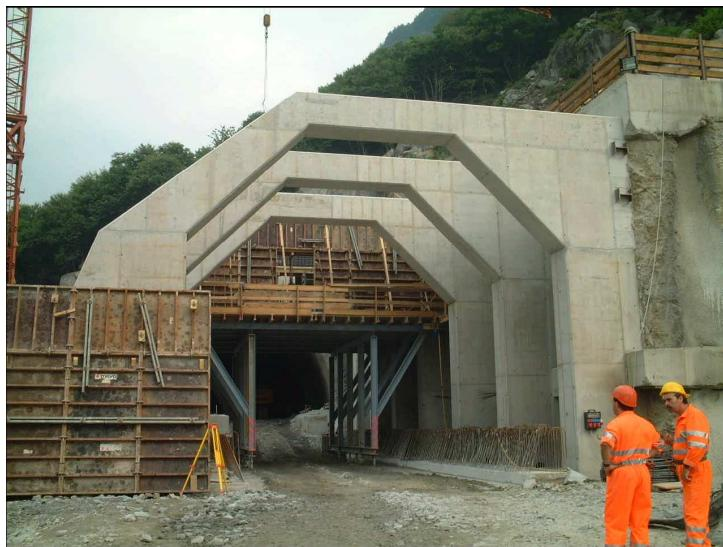
Figure 4: Support Buttresses at the south portal of the new Alptranist Gotthard tunnel
