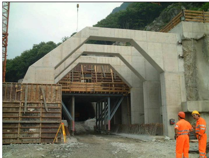
Figure 4: Support Buttresses at the south portal of the new Alptransit Gotthard tunnel
