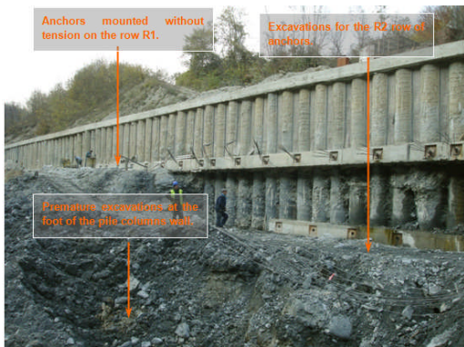
Fig. 2 The state of the works at the moment of taking over the project by TUCEB. Anchor installation
