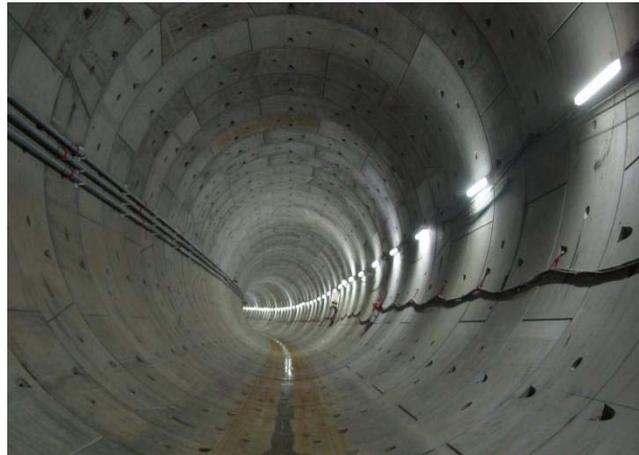
**Figure 2** The lining of the tunnel is formed by a continuation built up of the rings
