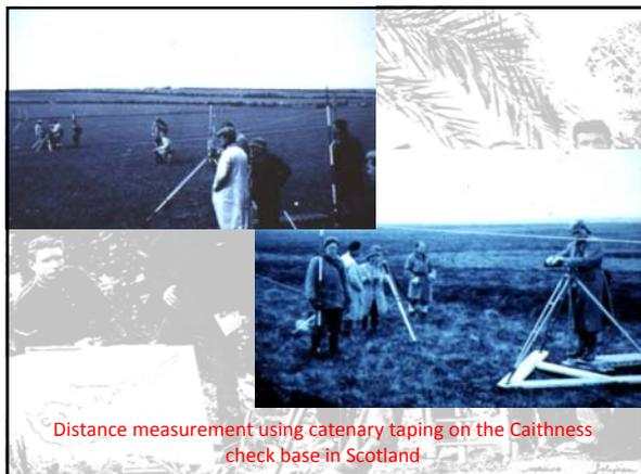
Distance measurement using catenary taping on the Caithness check base in Scotland
