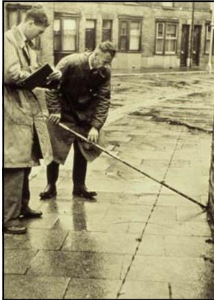
Chain survey in the Ordnance Survey, using the method of rectangular off-sets to survey detail. This was based on a 3<sup>rd</sup> order triangulation network, with triangles with side lengths of about 2,000 metres. The method was very time-consuming, but used very simple equipment.
