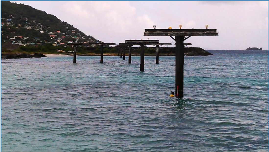
Figure 2.4 – Tide gauge being installed at Adams Bay, Bequia Photo: M. Sutherland (2012)
