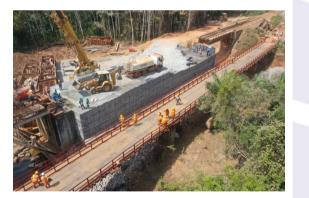
Rail Track Rein statement Precise elevation corrections of ±4cm restored operational functionality.
