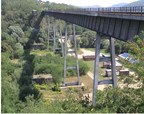
Fig. 2: View of the viaduct
