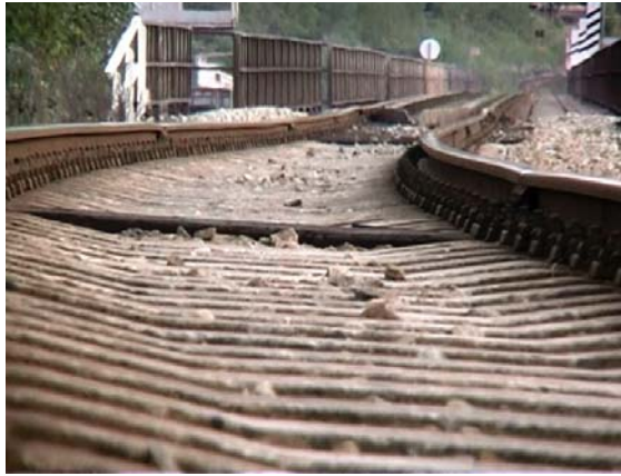
Fig. 1: Distortions of Rail Geometry
