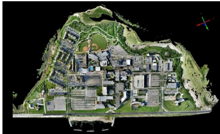
Figure 12: 3D point cloud of TAMUCC campus created from imagery taken using Sensefly eBee.
